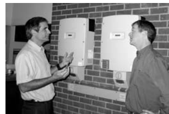
Dave Brennan, City Manager, and Sam Pierce, Mayor, in front of City Hall’s two new solar electric inverters.
